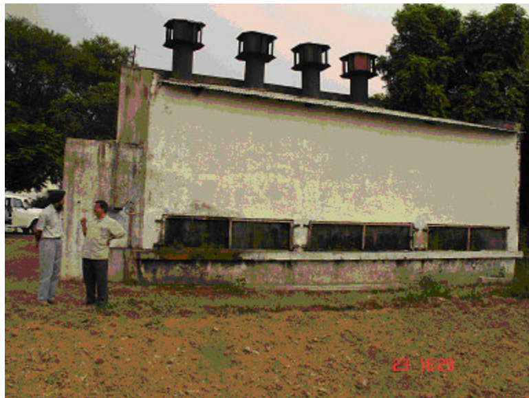
Evaporatively cooled storage structure of 20 tone capacity for short term storage of potatoes
